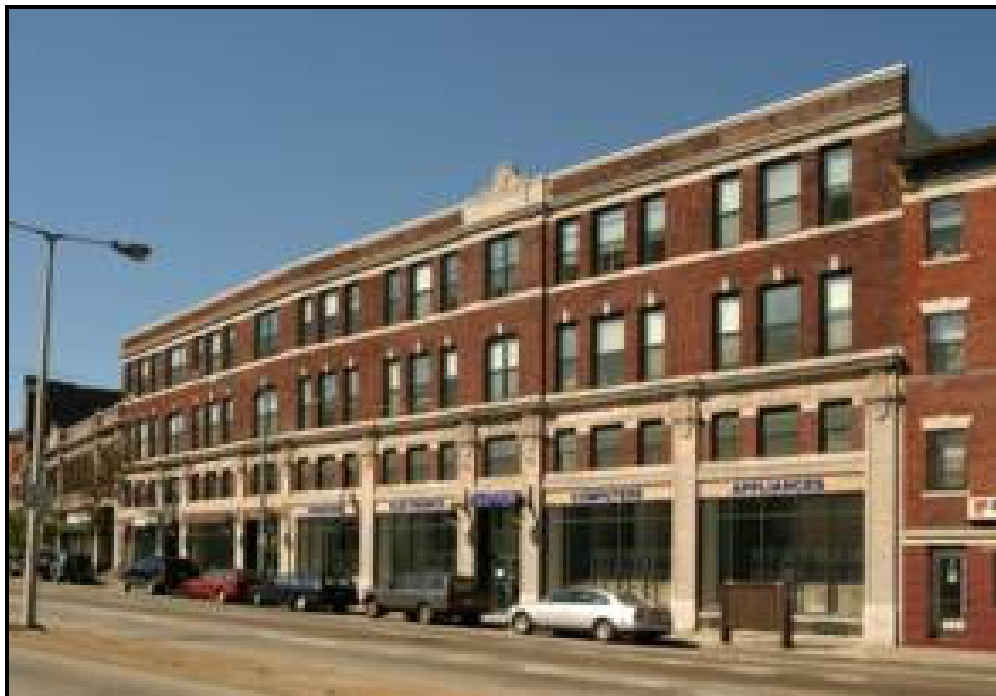
Entrance on Columbia Road
